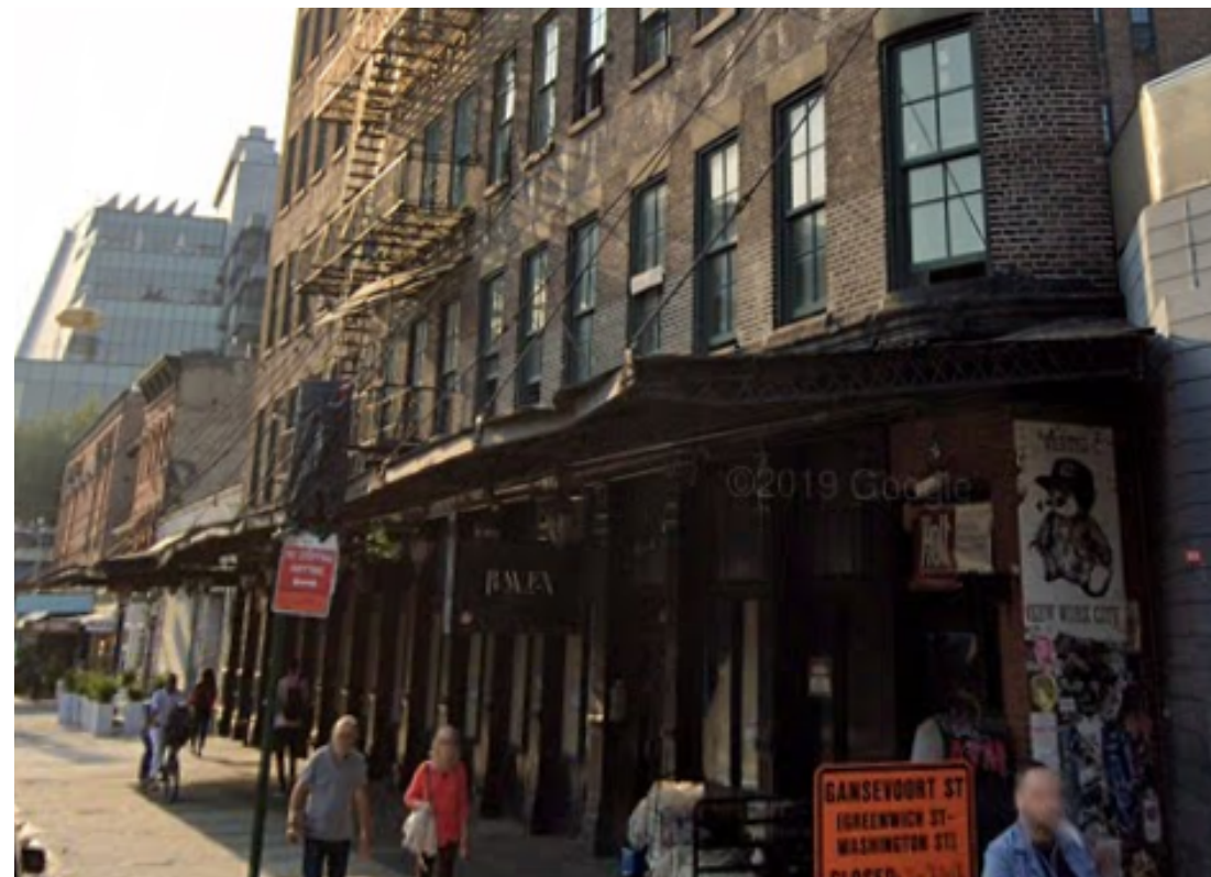
2017: Looking west on Gansevoort Street prior to the start of renovation
